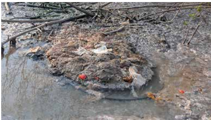
Effluent pouring out of the holding chamber serving the Grey Rock Estate.
