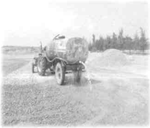
Water sprinkling on Roads
