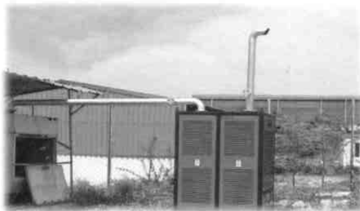
Retrofit Equipment at DG sets
