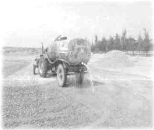
Water sprinkling on Roads
