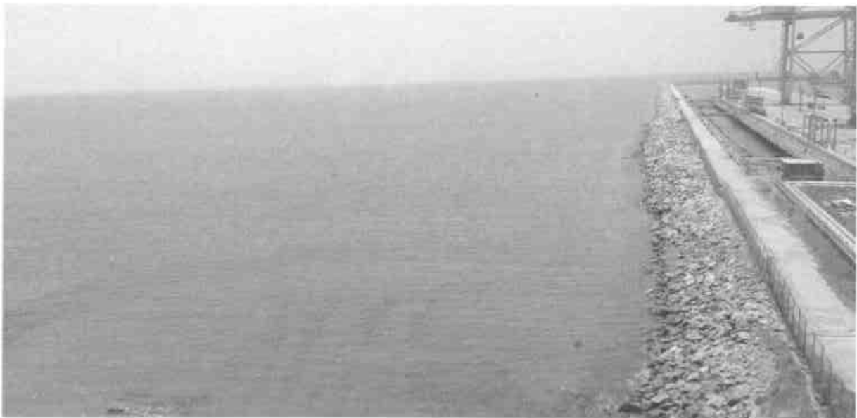
Fig. Distance between Northern Breakwater and Intake of CWDL
