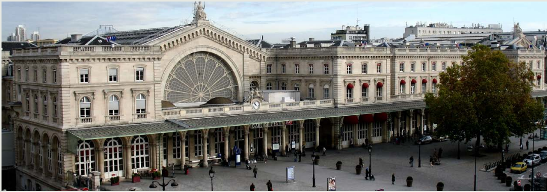
Historic central city station: Gare de l'Est, one of the six large terminal stations in Paris.
