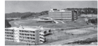
Completed Basic Research Laboratories (1962)
