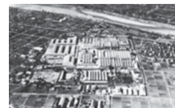
A bird's-eye view of Aichi Plant (1952)
