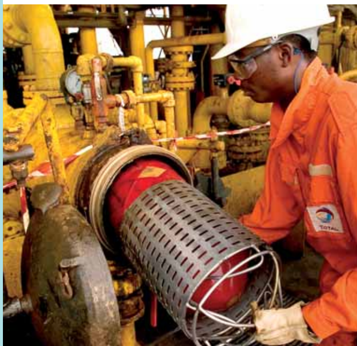
Congo: on the Sendji platforms, the low-pressure gas lines are cleaned out, or "pigged", every week.
