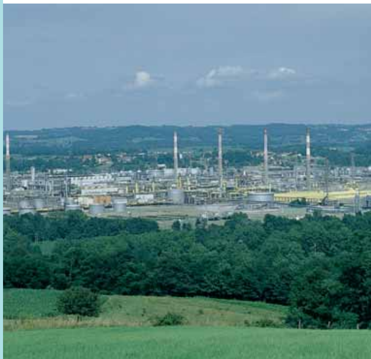
France: the gas treatment plant at Lacq
