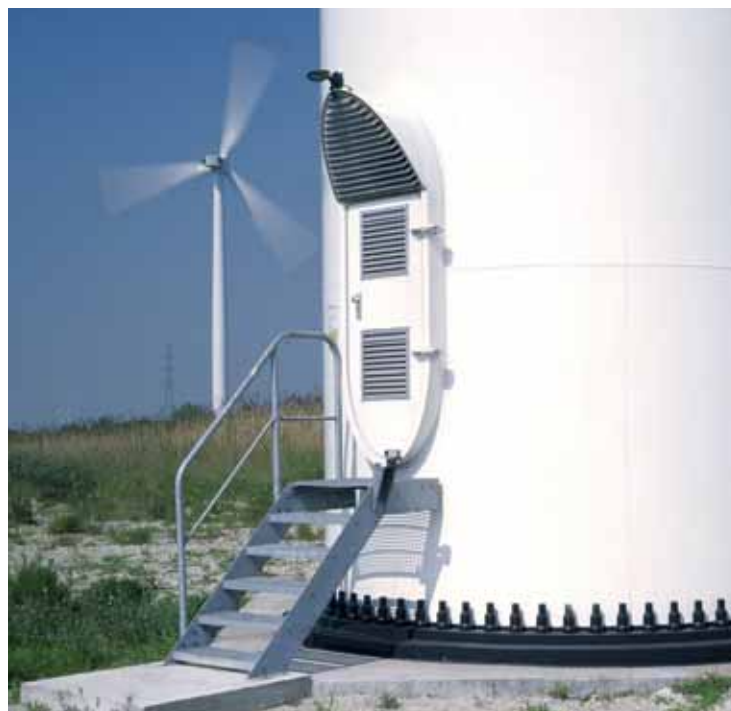
France: the wind farm on the Flanders refinery site at Mardyck, near Dunkirk, has five turbines with a total installed capacity of 12 MW.
