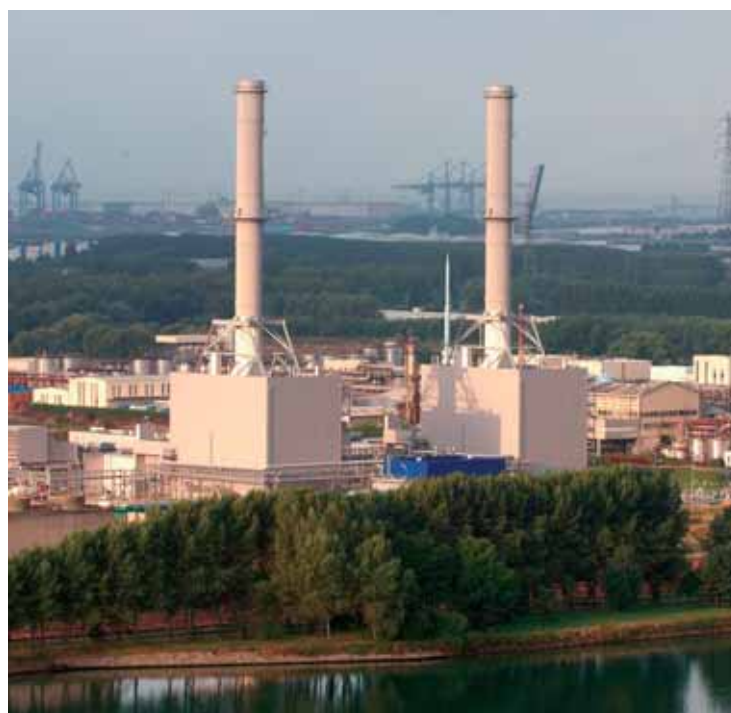
France: the cogeneration unit of the Gonfreville refinery
