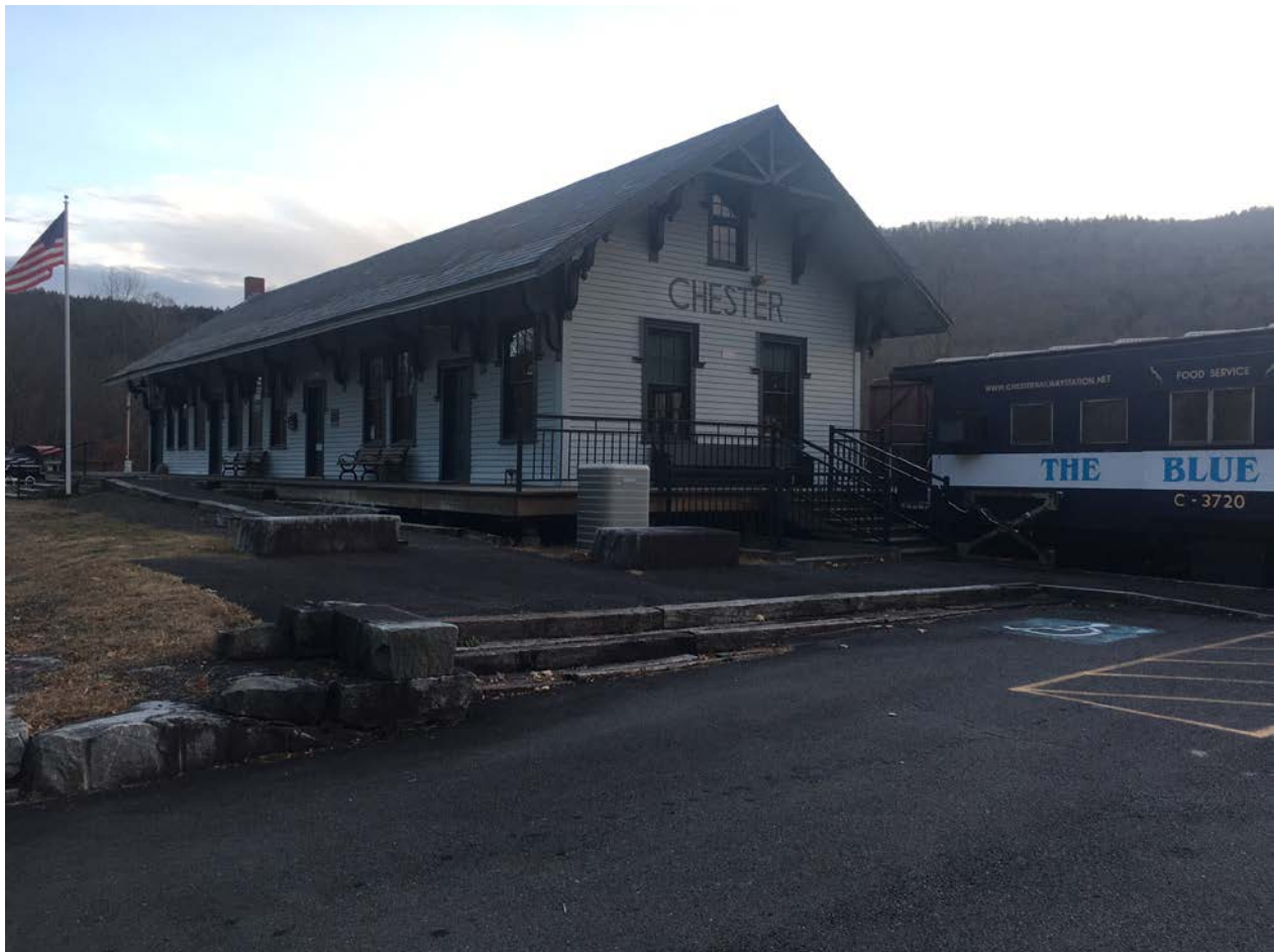
The old Chester railroad station is a visual reminder of the town's historical status as a railhub for the region.
