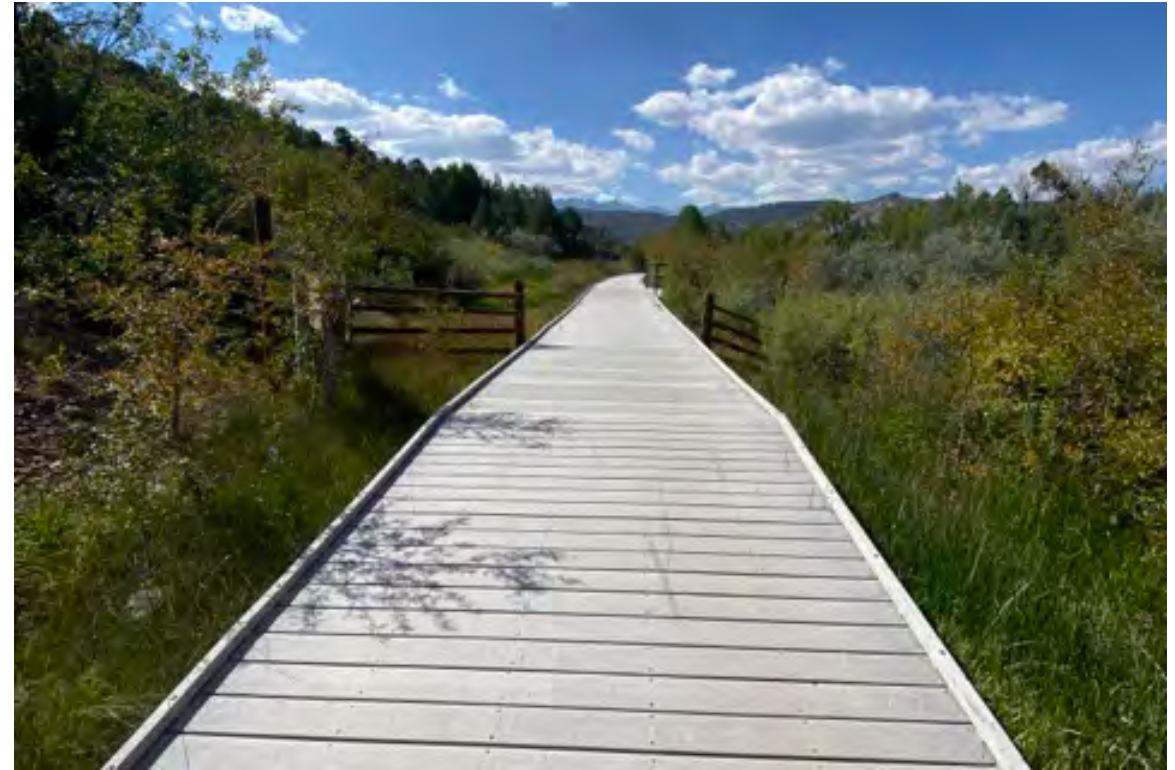
Photo 10: Existing constructed boardwalk over wetlands on BLM property.
