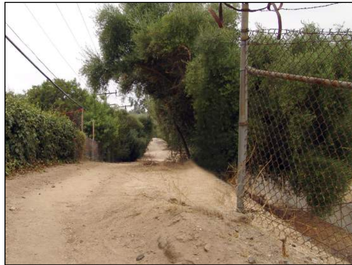
Figure 4.3.17-1 Chain Link Fence with Vegetation
