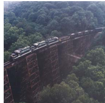
PAL train crossing a PAL high trestle bridge near Muldraugh, KY, one of the longest curved truss bridges in Kentucky.
