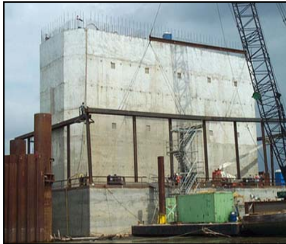
Figure 4-5. Greenville Bridge Pier 37
