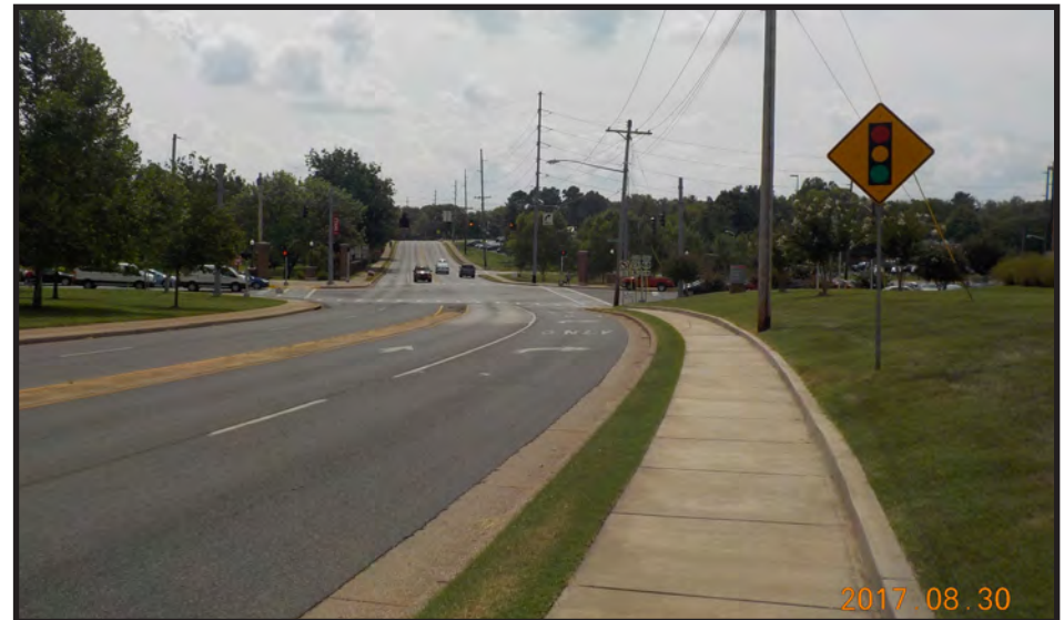
Photo 24: US 68X and US 231X intersection east junction from University Boulevard (US 68); facing southeast.
