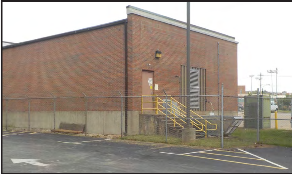
Photo 13: Western Kentucky University Supply-Services Out-building; field identified potential hazardous materials site; "Hazardous Waste" placard posted on door; facing northeast.
