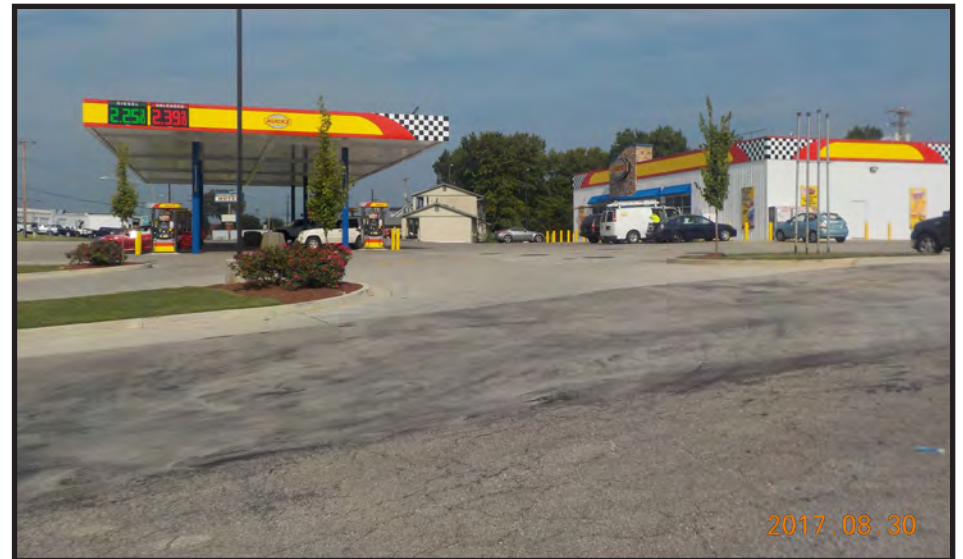
Photo 8: Huck's #395 gas station, UST record site (active), 306 Morgantown Road; potential hazardous materials site; facing northwest.
