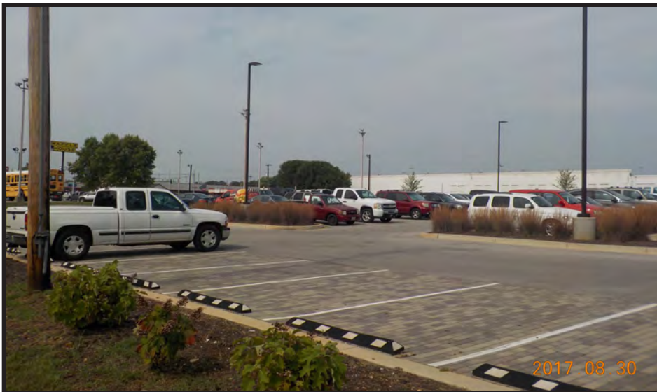
Photo 11: Representative view of a former (non-active) UST site; WKU Park & Ride, 1840 Russellville Road; potential hazardous materials concern site; facing west.
