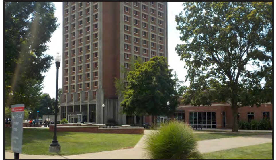
Photo 18: Sensitive noise receptor (Category B), Pearce Ford Tower residence hall and food court on Western Kentucky University campus; facing south.
