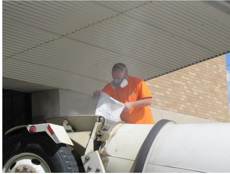
Figure 5.1 – Adding calcium hydroxide to the mixing truck
