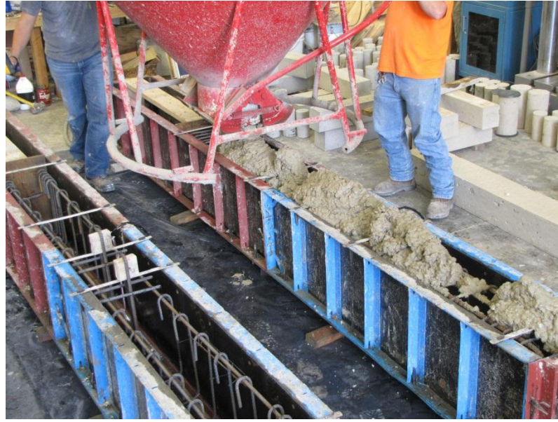
Figure 4.13 – Placement of concrete into beam forms
