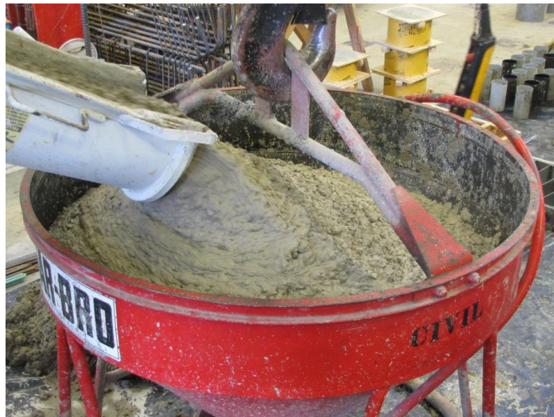
Figure 4.12 – Concrete bucket being filled with fresh concrete
