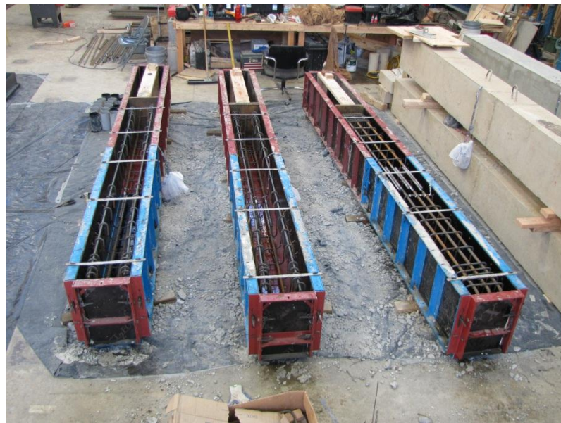
Figure 4.11 – Reinforcing bar cages in beam forms
