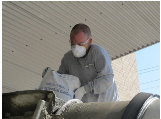
(b) Adding calcium hydroxide
