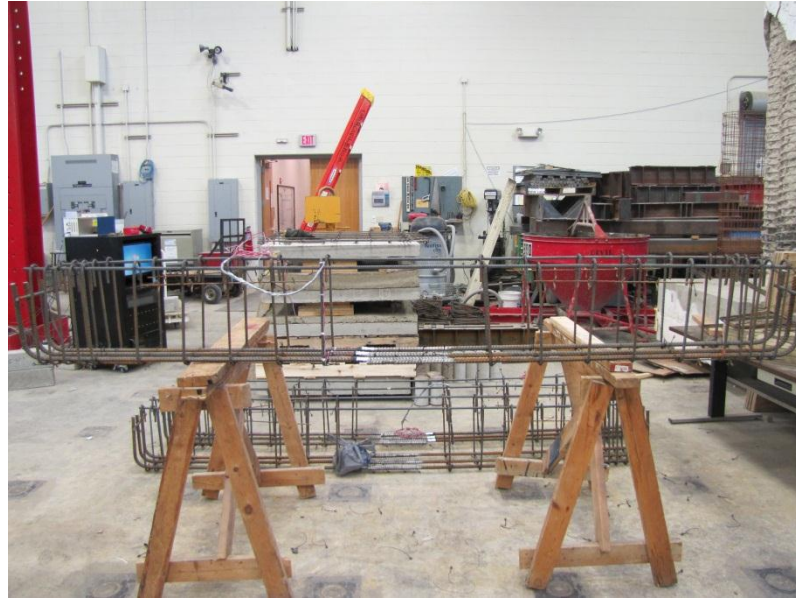
Figure 4.9 – Finished reinforcing bar cage
