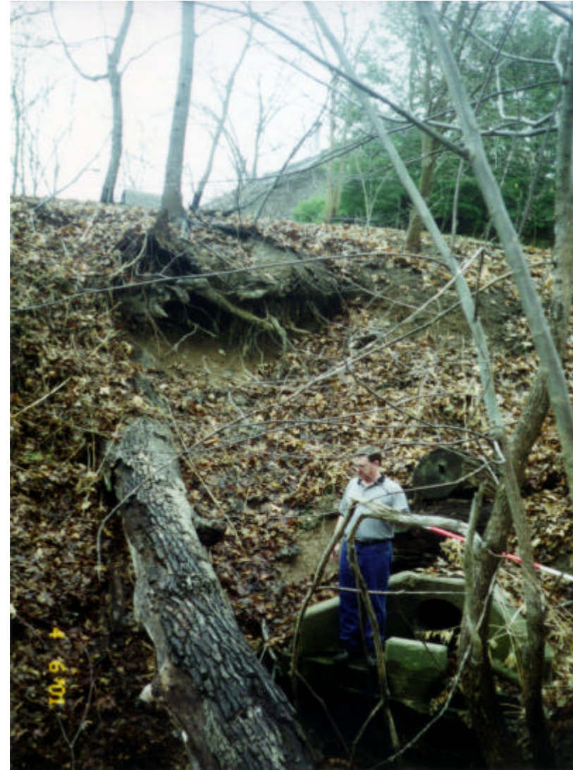
Photo 4 Study Area #12 - Sleepy Hollow Road - Looking US and to the LT of SS outlet. Note tree life in jeopardy due to slope failure. (0_pic23.jpg)
