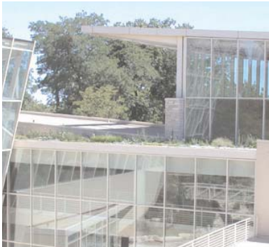
Figures 36 & 37 (below). Images show green roof technology. Photograph of green roof pilot project at the Peggy Notebaert Nature Museum (Chicago, IL).
