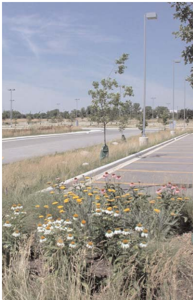
Figure 44 (above). Photograph shows bioswale in a parking lot. Pavement slopes towards area planted with deep and fibrous rooted native vegetation (Tellabs Corp. Naperville, IL).
