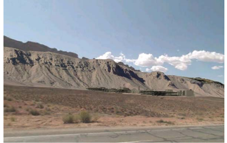
SOUTH WEST VIEW FROM HIGHWAY 191
