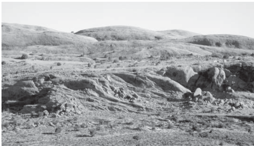
Figure 9. Example of moderate rock-fall-hazard area, where Sand Flats Road traverses Navajo Sandstone "slick rock" southeast of downtown Moab. Rock falls occasionally occur in these areas, but the relative lack of rock-fall sources and the generally limited travel distance of rock-fall boulders results in a lower hazard than in other rock-fall-hazard areas (see figure 8).
