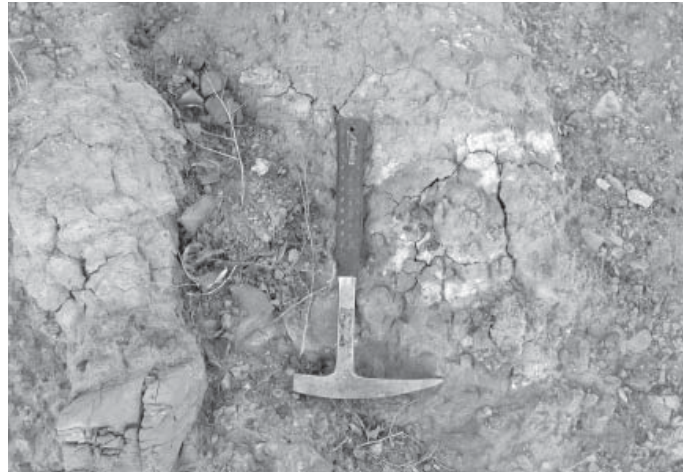
Figure 4. Fractures formed by shrinkage in expansive clay in a mudstone interbed of the Chinle Formation. Outcrop exposed in cut at base of slope east of downtown Moab.
