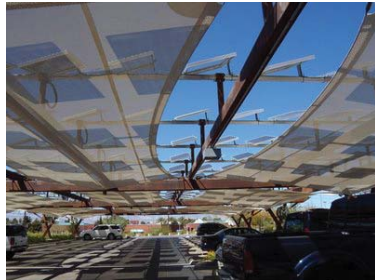
SHADED PARKING STRUCTURE. SPRINGS PRESERVE; LAS VEGAS, NV
