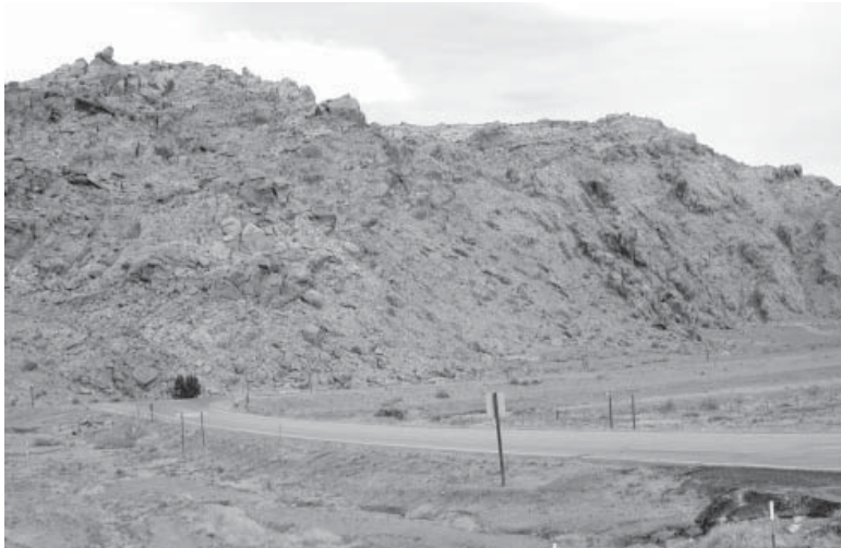
Figure 10. Highly fractured Navajo Sandstone exposed at the northwestern end of Moab-Spanish Valley, at the intersection of Utah Hwy. 279 (foreground) and U.S. Hwy. 191 (at base of slope). Fractured rock such as this poses a variety of problems for development.
