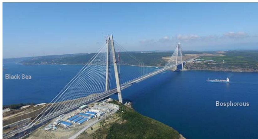
Photo 2. Yavuz Sultan Selim Bridge exit of the Istanbul Strait ( sabah.com.tr )
