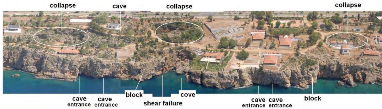
Figure 11. Cave and cave collapse features of the tufa coastline.
