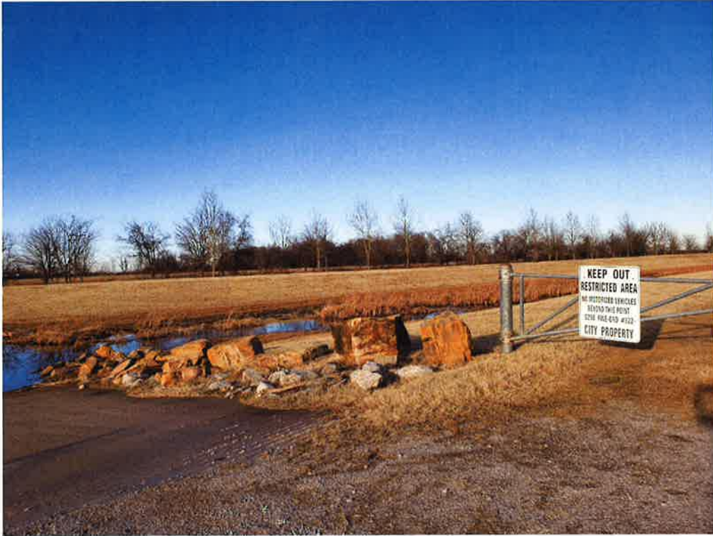
Looking northeast at Bixby Creek crossing
