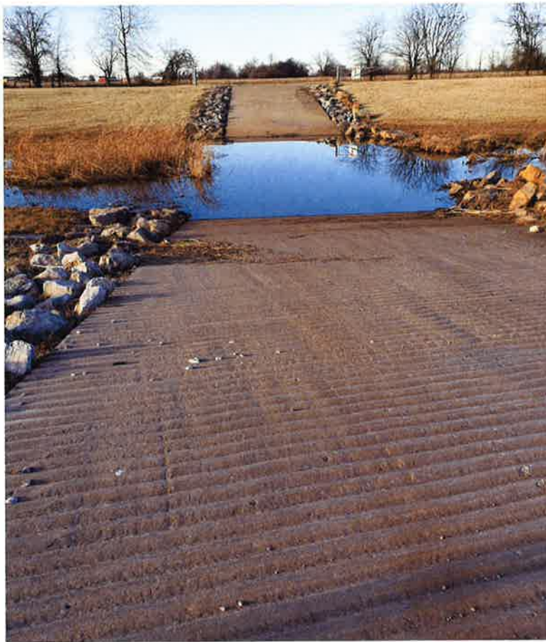
Close-up of creek crossing
