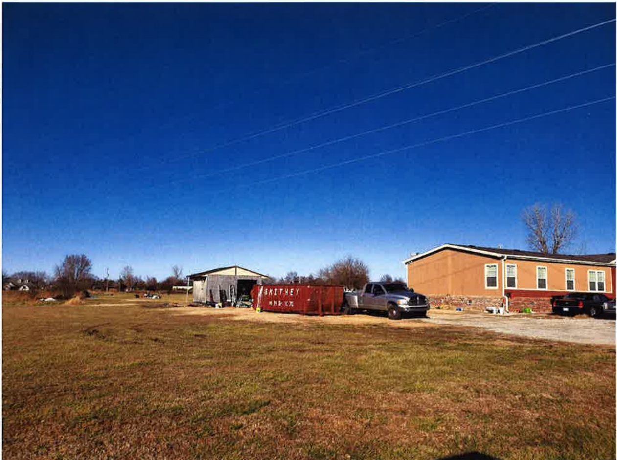
Looking northeast at subject property from E. 177th St. N.
