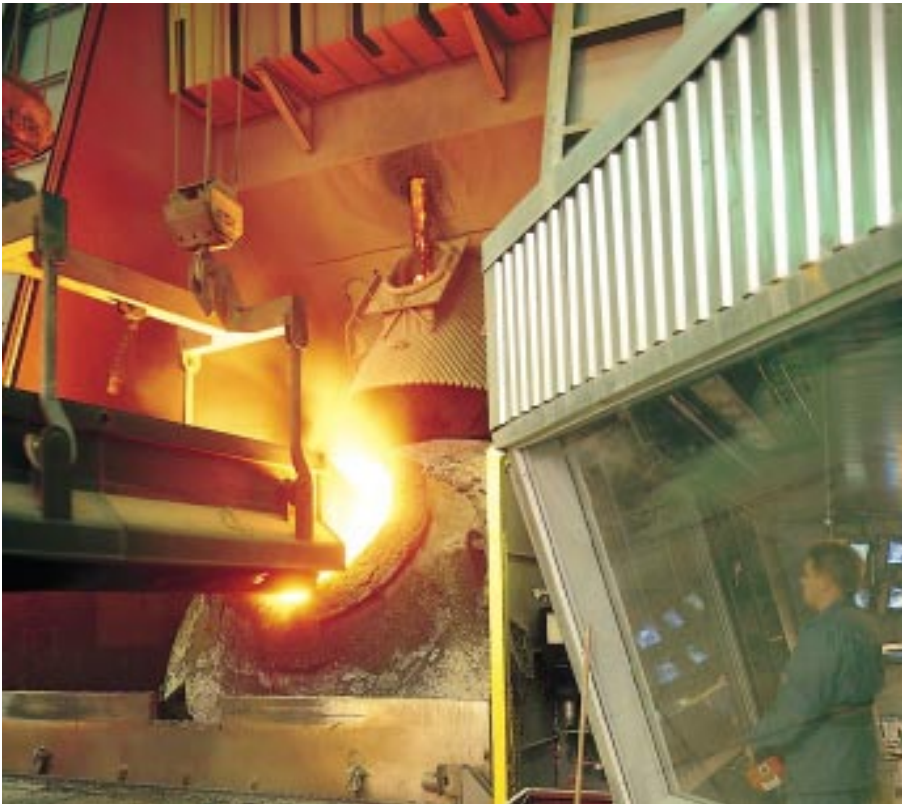
The ferrochrome converter enables the steel melting shop in Tornio to charge almost all ferrochrome in liquid form. Scrap, an important stainless steel raw material besides ferrochrome and nickel, is being charged into the converter.
