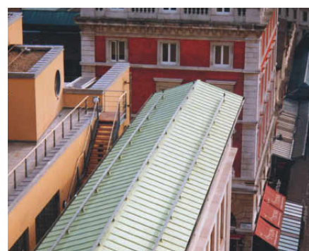
The Outokumpu developed, Nordic Green pre-patination method was used in the re-roofing of Covent Garden in London in 1999.
