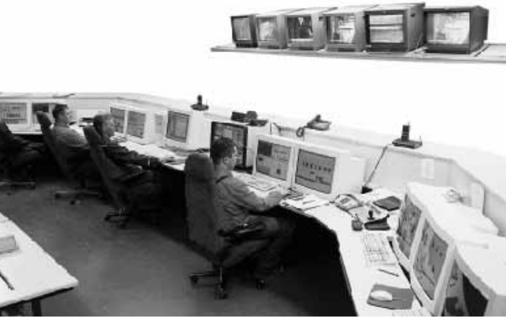
The Kokkola expansion project was completed at the end of 1998. During 1999 production ran at full capacity, 225 200 tonnes. Janne Marttila (left), Juhani Taivassalo and Veikko Erikkilä oversee the process in the new central control room.
