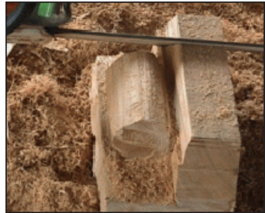
Figure 94. A new runner was sculpted to replace the rotten wood.
