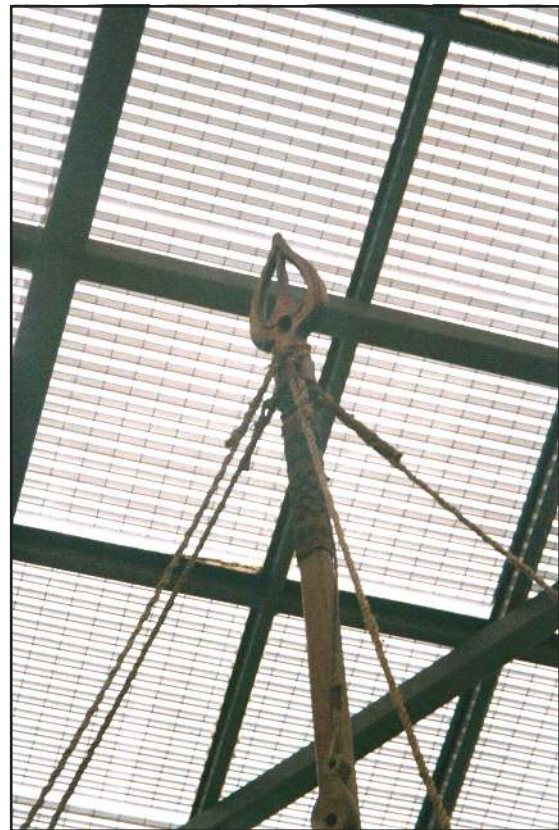
Figure 20. Top of mast with four shrouds (Nadi Airport).
