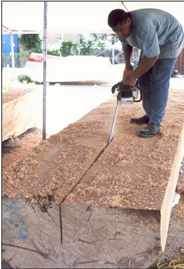
Figure 51. Making central cut in order to begin hollowing out the log.
