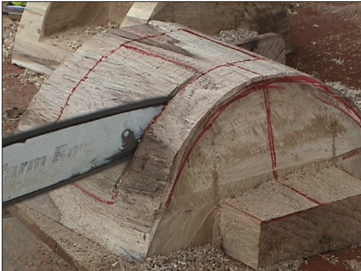
Figure 118. Two wedges were cut out to make the step for the foot of the mast.
