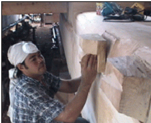
Figure 95. New runners were placed in position.
