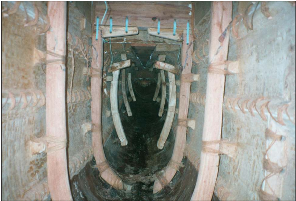
Figure 84. View into the prow from roughly 25 feet back from the prow tip. The two sets of ribs in foreground were made of Calophyllum vitiense and three sets of ribs up in the prow were made of Agathis vitiensis wood.
