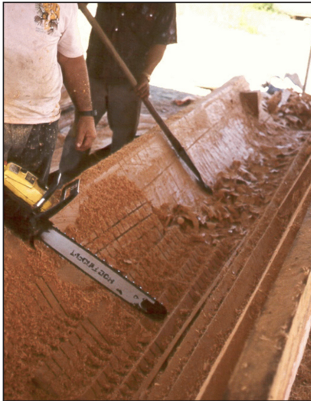
Figure 56. Crosshatching with the chainsaw and chisel work.
