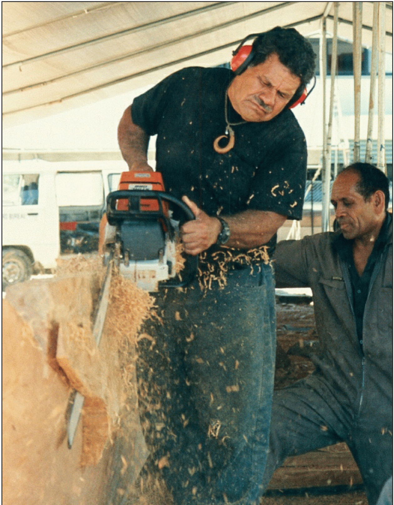
Figure 64. The strake exterior surface was trimmed to be flush with the hull segment.
