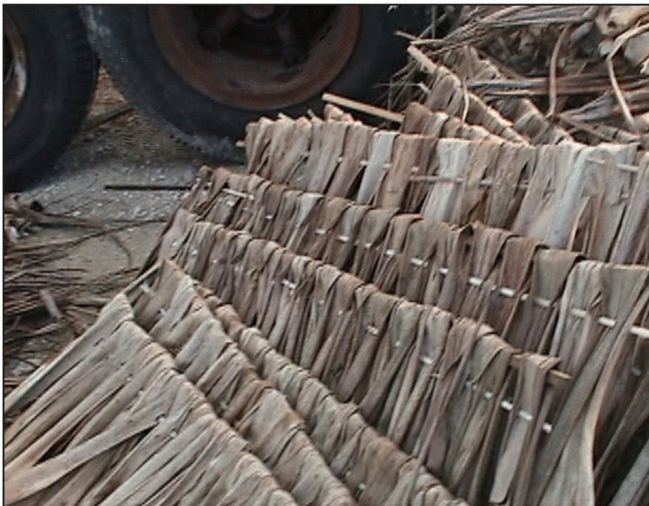
Figure 116. Rows of pandanus leaves pinned together with skewers for roof of fale.
