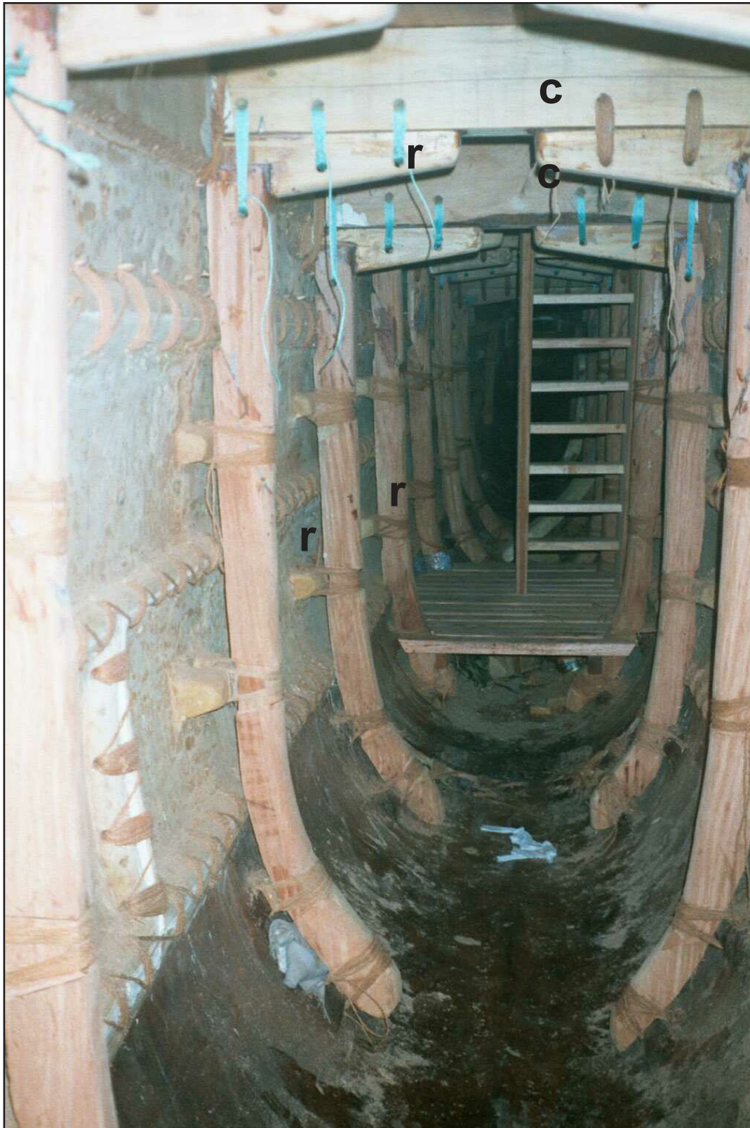
Figure 83. Ribs (r) are shown here connected to the crossbooms (c).
