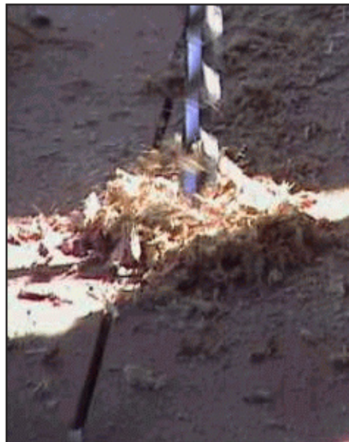
Figure 103. Holes were drilled for lashing the deck planks to the crossbooms.
