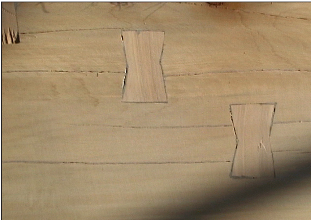
Figure 143. Butterfly plugs gripped the wood across the grain to hold it together.
