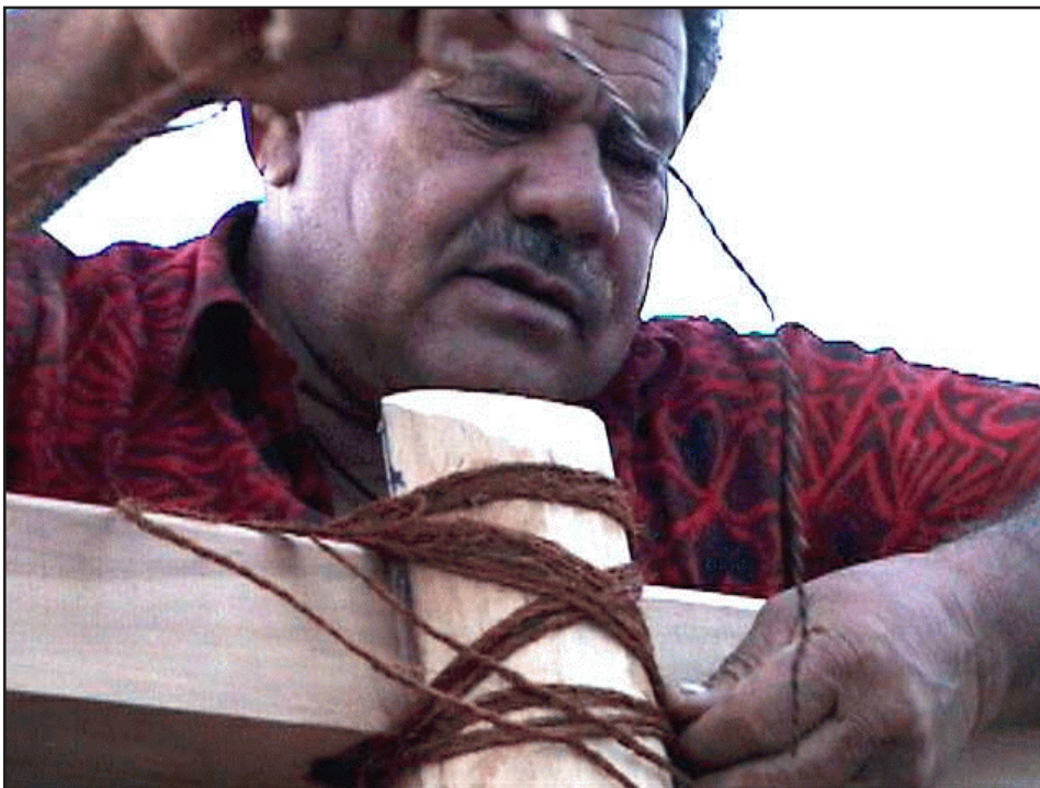
Figure 112. Lashing post on windward side of lookout deck to cross post.
