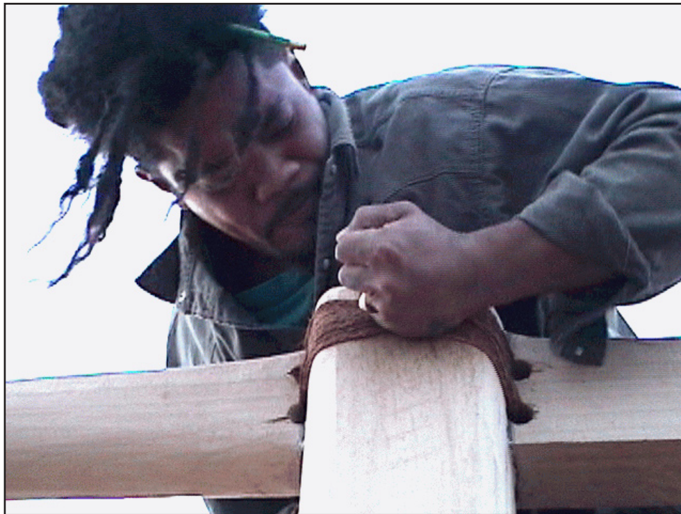
Figure 114. Lashings were made as tight as possible.
