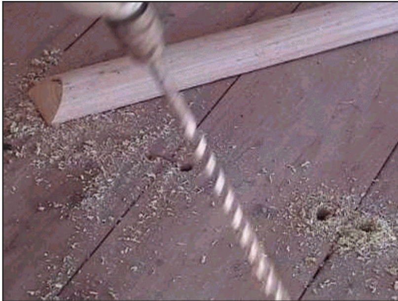
Figure 104. Holes were drilled near the edges of the planks..
