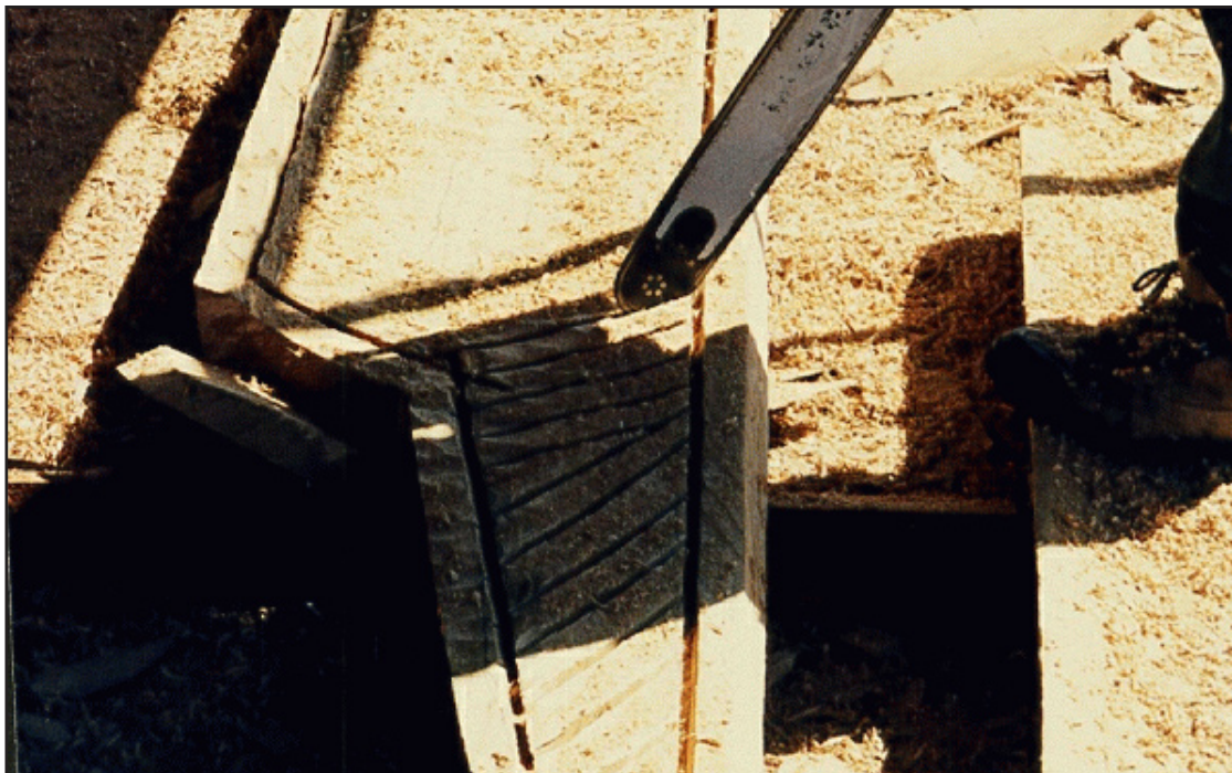
Figure 70. The inner surface of the strakes were scored with the chainsaw.
