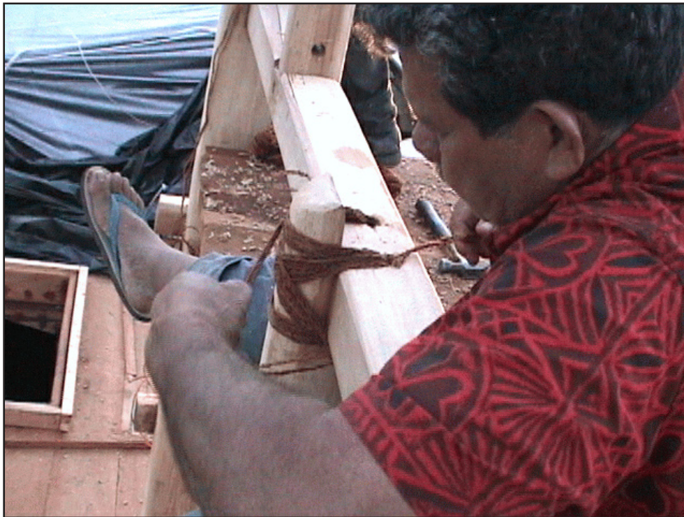
Figure 113. Lashing through holes drilled on either side of the support post.
