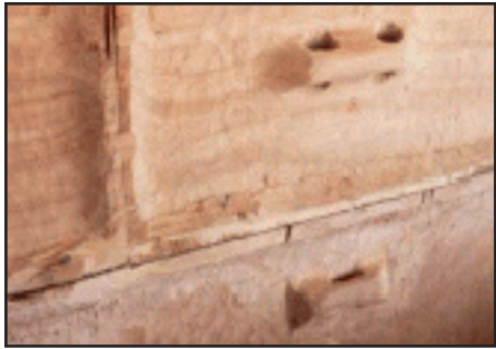
Figure 75. Comb cleats lined up between adjoining strake and hull segment.
