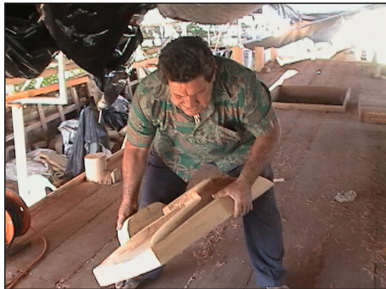
Figure 123. Placing one of the two yard grooves for the middle of the deck into place.
