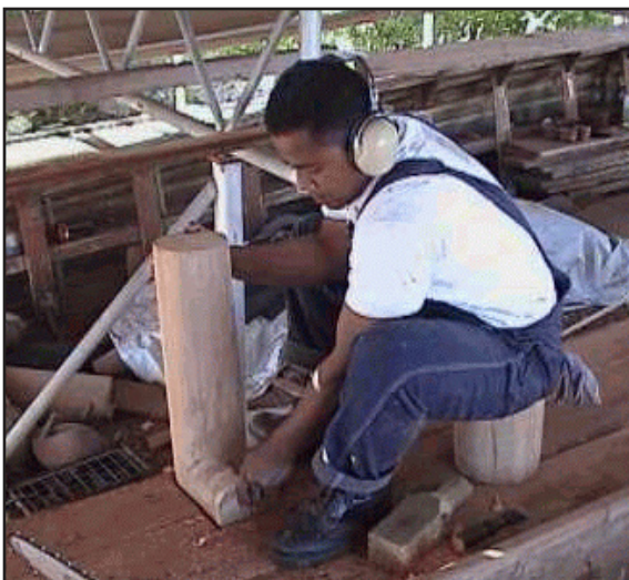
Figure 98. Placement of yard rail post.
