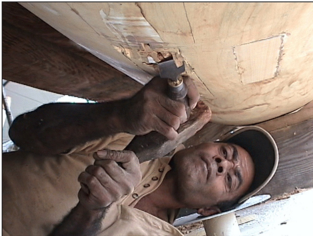
Figure 137. Removal of the rotten material was done with chisels.
