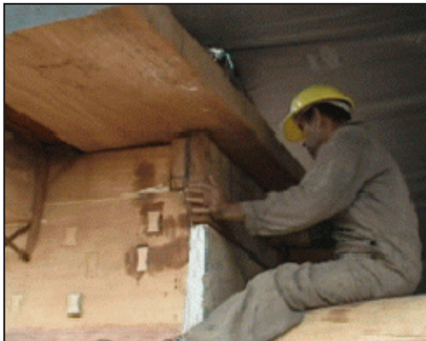
Figure 90. Viliami Kolomatangi placed the last piece of the breakwater into position.
