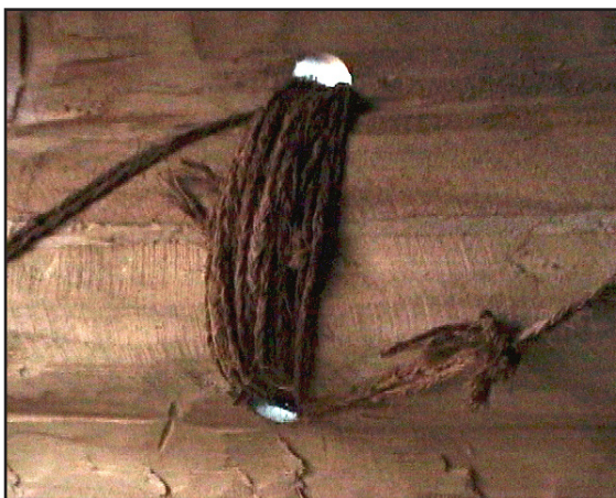
Figure 81. Interior view of a lashing between the second strake layer and washstrake layer. 1" holes which were drilled through hull to the exterior. The batten was on the exterior side and bound to the hull by this lashing.
