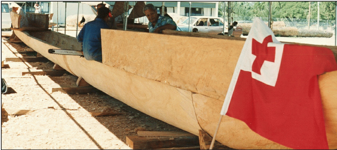
Figure 59. Hull segments 2 through 4 were laid out horizontally along ground.
