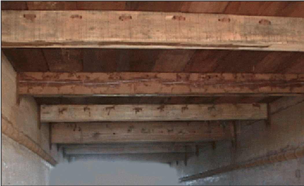
Figure 106. This view underneath the deck shows nearly all the crossbooms and both hulls. Note the deck lashings visible on the crossbooms.
