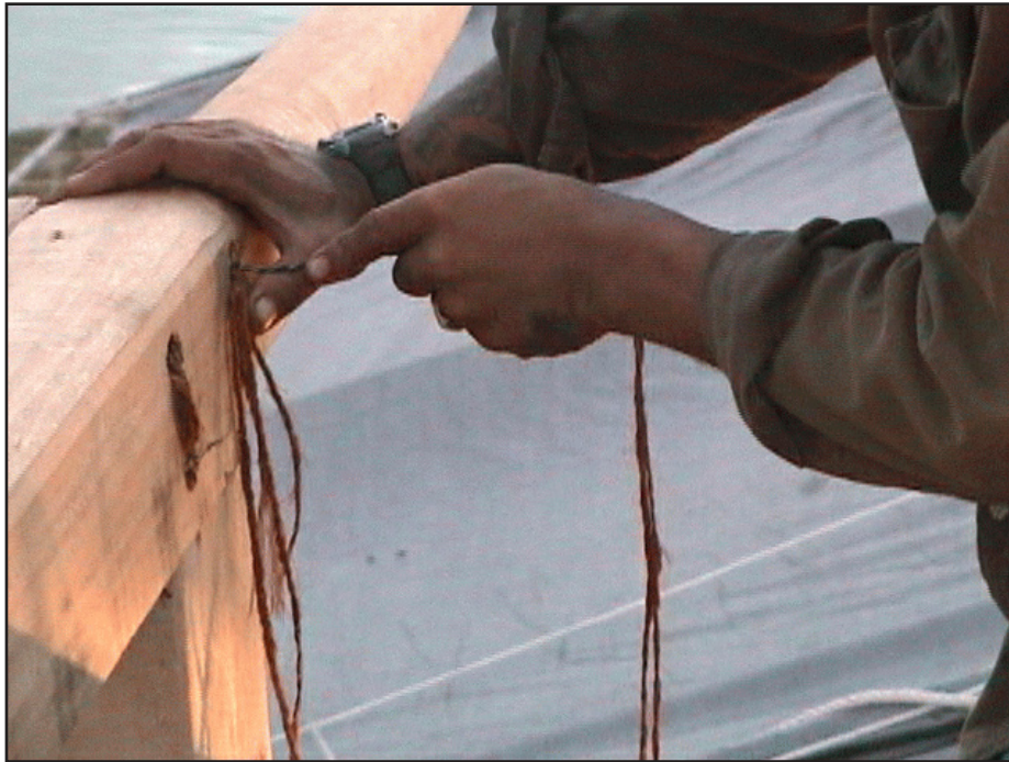
Figure 115. Two pairs of holes on back of the cross post where the wire needle passed the lashings through..
