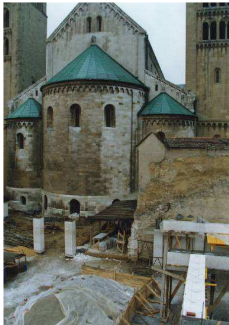
Fig. 4. Construction site of the Cathedral Museum in the former moat
