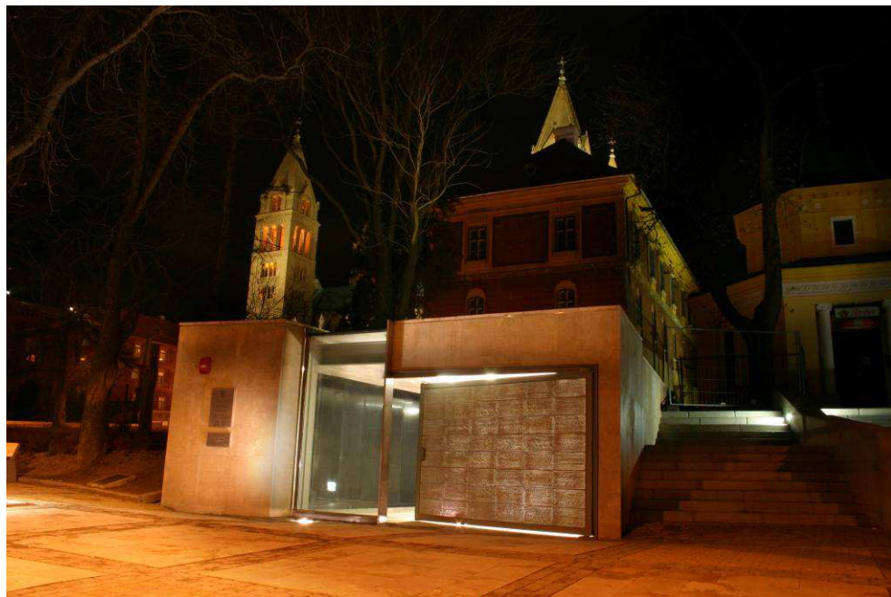
Fig. 14. The entrance of the Cella Septichora Visitors' Centre
