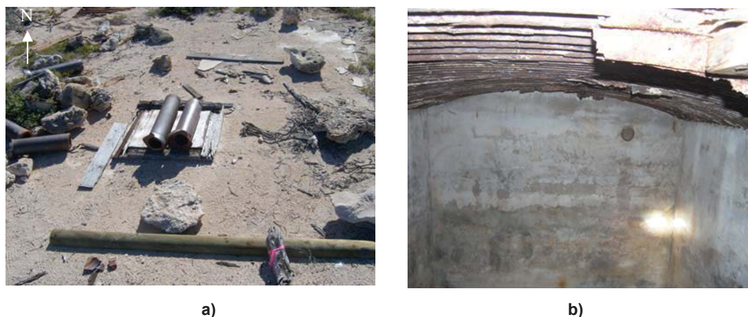
Figure 9.25. a) Close up of lid to underground water cistern and b) inside view of the cistern (right). No water was present in tank at time of archaeological surveys. Note: the treated pine log present in foreground of photo is recent and was brought to the island by CALM in the 1990s.
