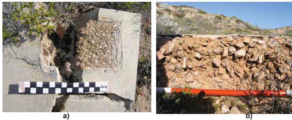
Figure 9.33 a) Photograph of the wooden beam imprint and b) cross section of the concrete pad on the outpatients building.
