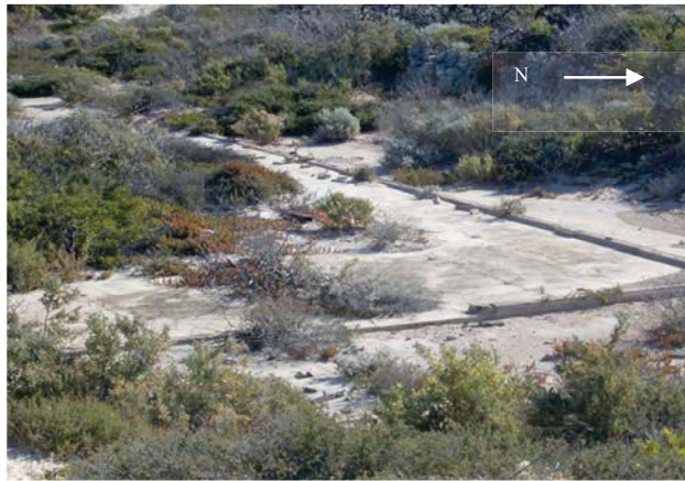
Figure 9.15. Concrete slab of ward structure on Dorre Island.
