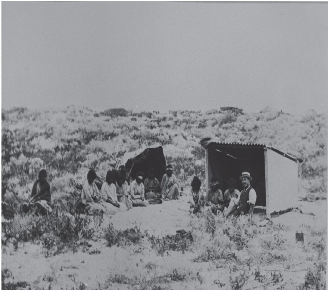
Figure 6.18. Female accommodation on Dorre Island, made of corrugated iron (Battye Library 21086P).
