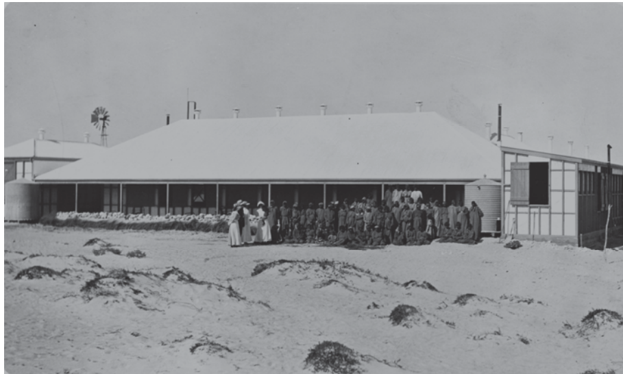
Figure 6.17. Examples of water collection and storage (windmill and water tanks to left of building) (Battye Library 3185B/22).
