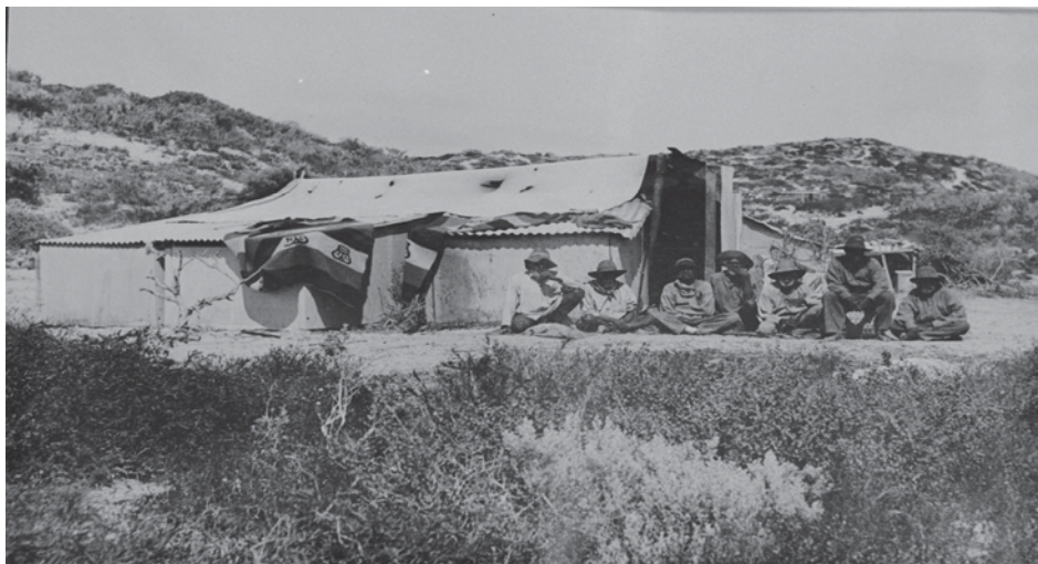
Figure 8.63. Historical photograph of Aboriginal accommodation on Bernier Island. Example of the corrugated iron structures that were provided during the scheme (Battye Library 21075P).
