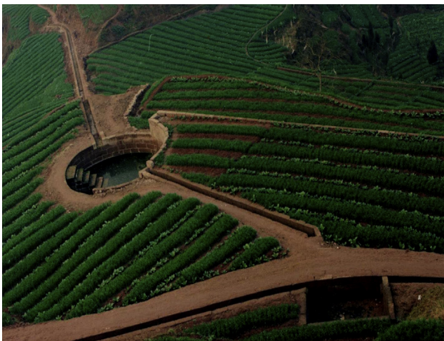
Figure 2.10 A rainwater catchment facility built in the middle of a field to catch runoff from intense summer rainfall events and used for supplemental irrigation later in the crop season. (For color version of this figure, the reader is referred to the online version of this book.)
