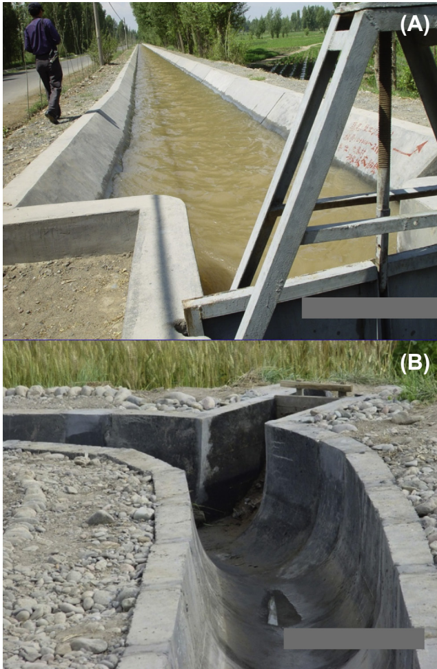
Figure 2.11 Improved water transportation systems: (A) a reinforced concrete main canal taking water to major distribution points, and (B) a “U”-shaped channel made from concrete blocks taking water to individual fields. (For color version of this figure, the reader is referred to the online version of this book.)
