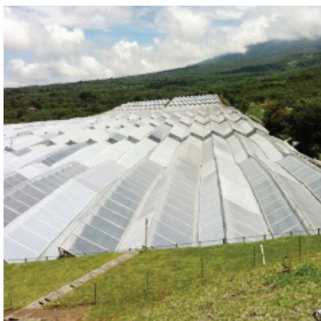
Fig. 2. Fully covered greenhouses with high roofs and the ability to vent hot air from the roof through insect screening. Photo: J. Bethke.
