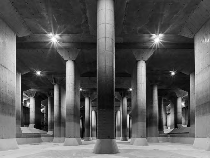
FIGURE 15.1. Water Chamber. Inside the 248,508 cubic feet water chamber, are five-dozen 60-foot high pillars, each reinforced by five hundred tons of concrete. Released under the GNU Free Documentation License.
