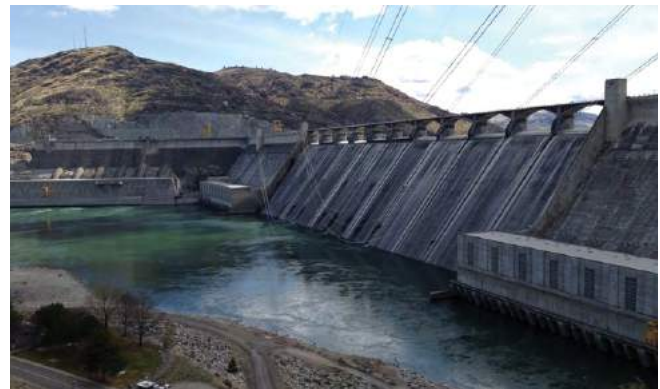
Grand Coulee Dam , Source: CRITFC
