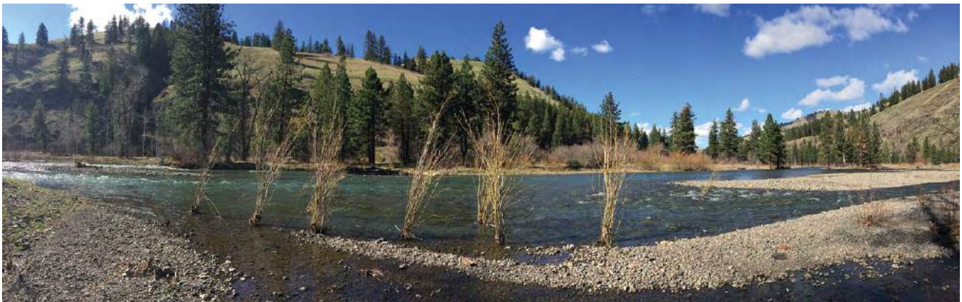
Meacham Creek habitat restoration project. Work done by the Conf. Tribes of the Umatilla Indian Reservation, Source: CRITFC
