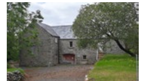
→ Significant redevelopment has been done to an important part of the Northwest's heritage.
