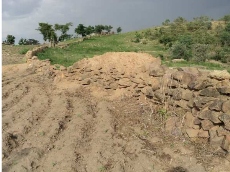
Figure 65: Gujimba walling system.
