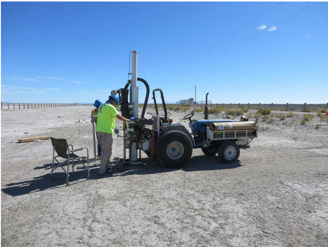
View east of coring work at BC3.
