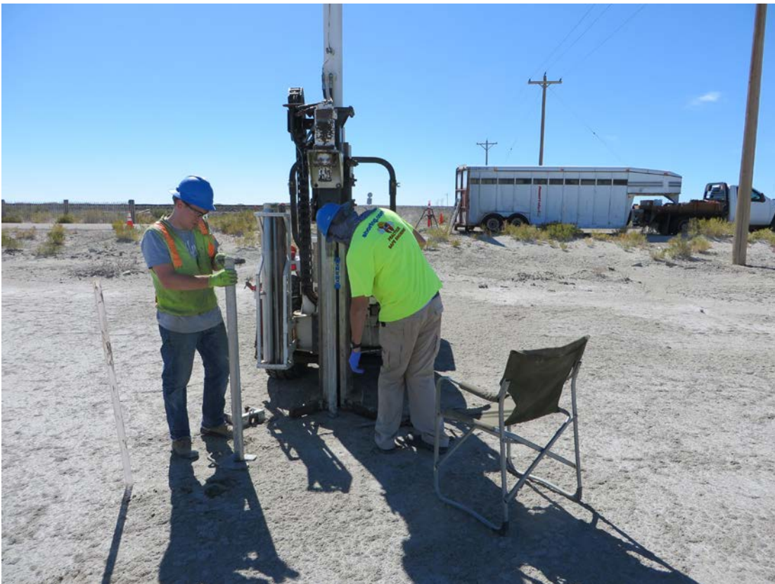
View south of coring work at BC3.
