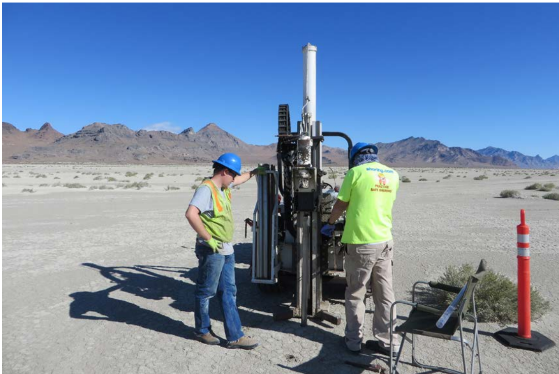
View north of coring work at BC2.
