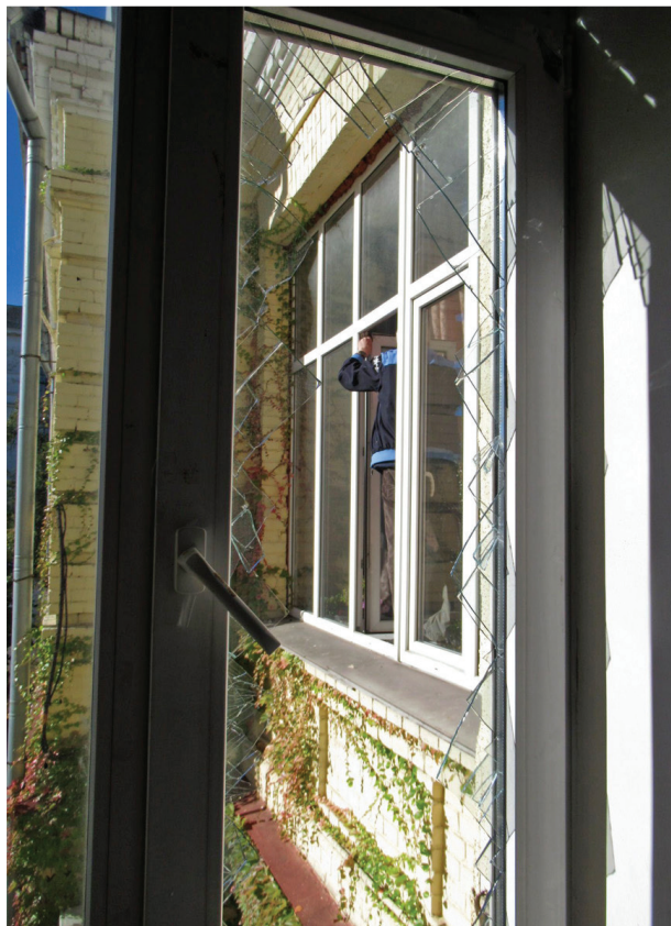
Fig. 4. Staff members of the Institute repairing the damaged windows
