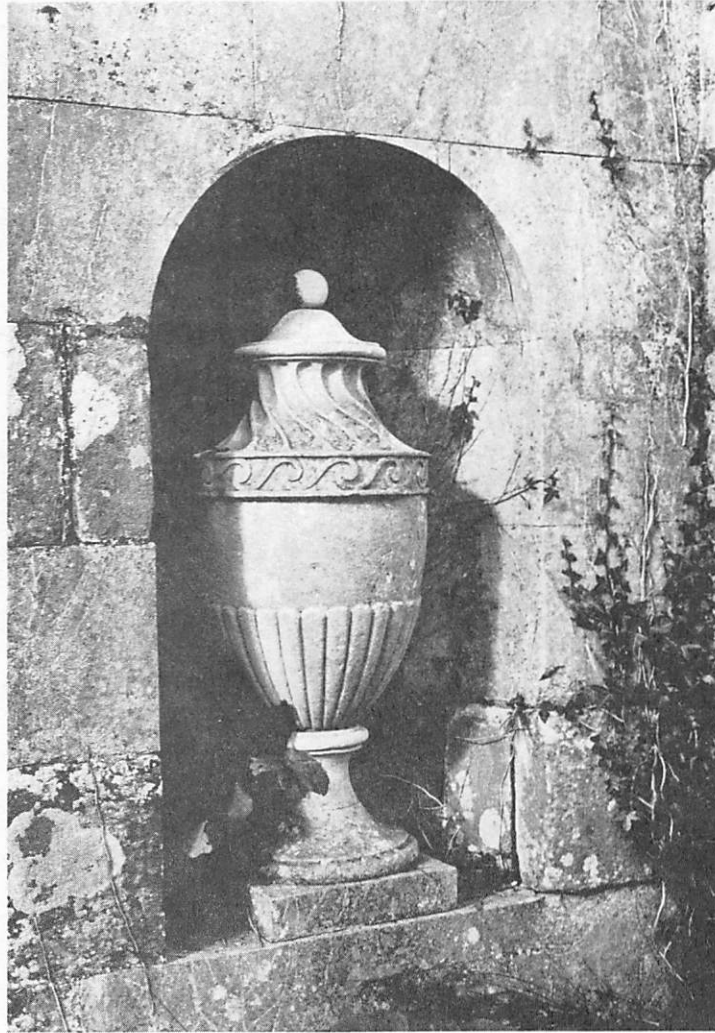
Urn designed by Robert Adam, Templeton Mausoleum, 1789 (No 41; photograph taken before restoration)
