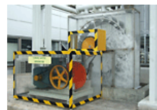
Hydropower utilizing cooling water from the plant
