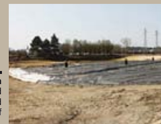
The former lagoon has been dried out and covered with a leakproof geomembrane.
