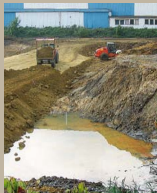
A new leak-proof storm basin has been created to collect rainwater.
