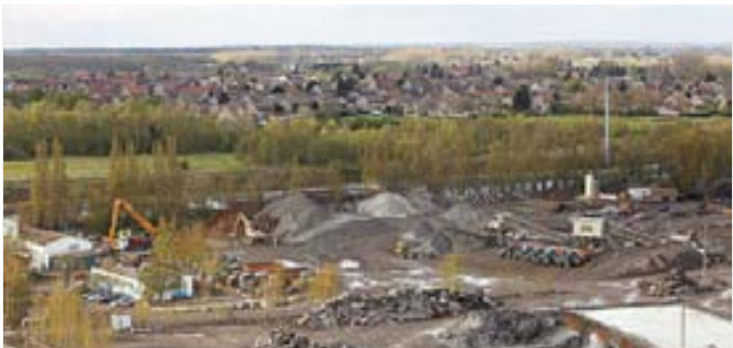
At Saint-Saulve, the slag produced by the electric arc furnaces is recycled by partner companies for road building and other uses.
