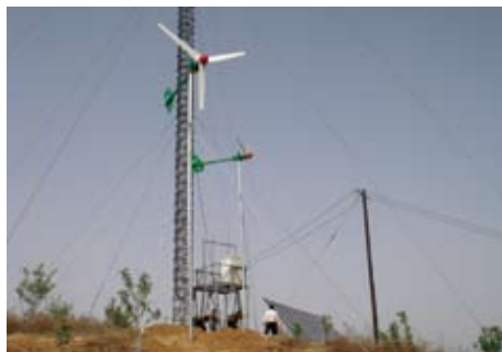
In Shaanxi, we introduced wind-solar hybrid power supply systems for base stations
