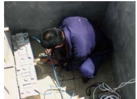
In Gansu, we installed batteries underground to reduce energy consumption
