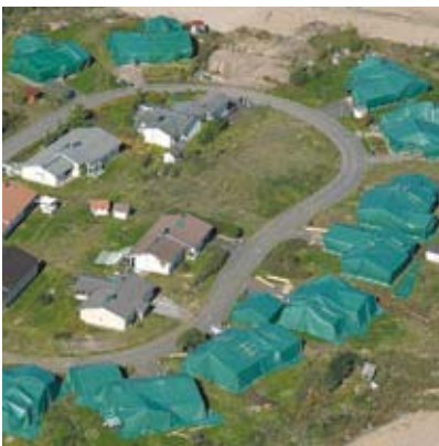
■ The soil in the residential area of Huhmarniemi was remediated in summer 2003. The residents moved elsewhere for the duration of the work and the buildings were covered. The contaminated soil in the plot area was removed and replaced with clean soil.
