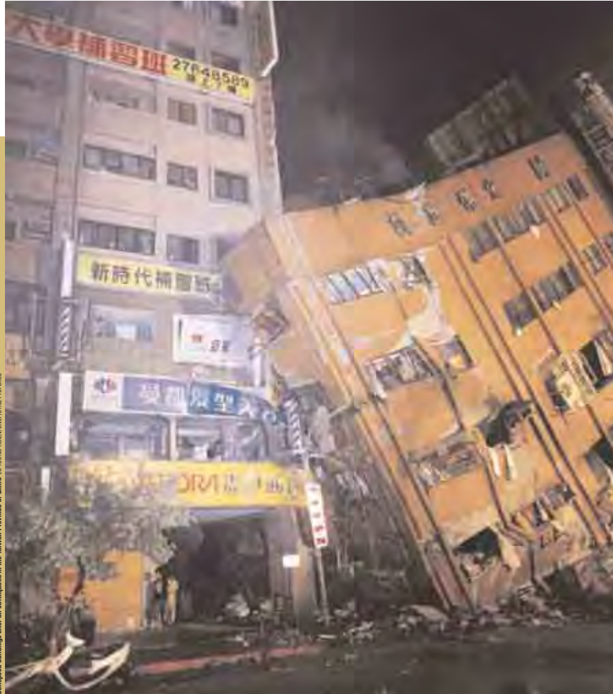
Collapsed buildings after an earthquake in the Taiwan Province of China. LO TSUNG HSEUNG/ISTOCK PICTURES
