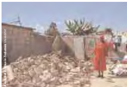
Demolition of a backyard extension.
