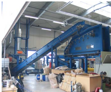
Figure 2: Pilot plant station for medium density fibreboard production
