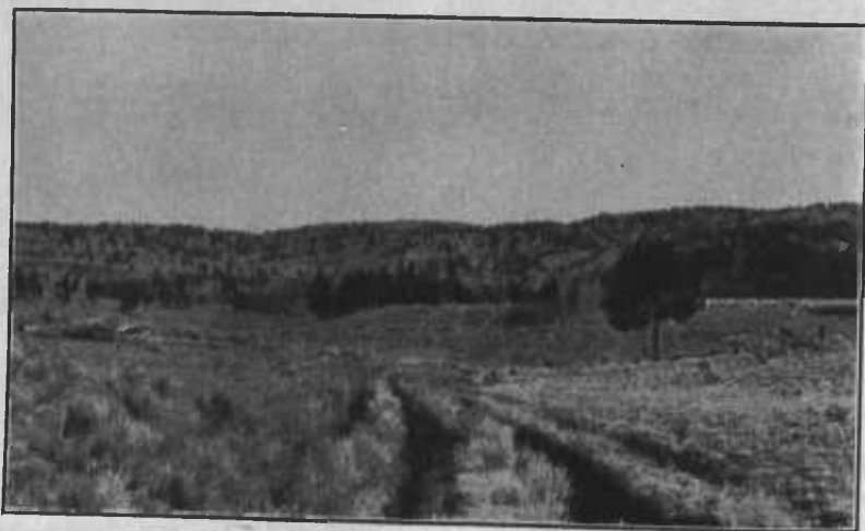
FIGURE 30.—Gullies follow the wagon wheel. Roads have been the direct cause of the beginning of destructive erosion in many drainage lines. Gully cutting has been invited, even on many modern roads, by inadequate road drainage and the concentration of floodwaters in culverts.
