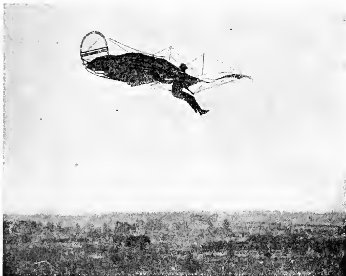
Otto Lilienthal in his single-plane glider. The swinging forward of his feet tends to turn the glider toward the ground, and increase its speed.
