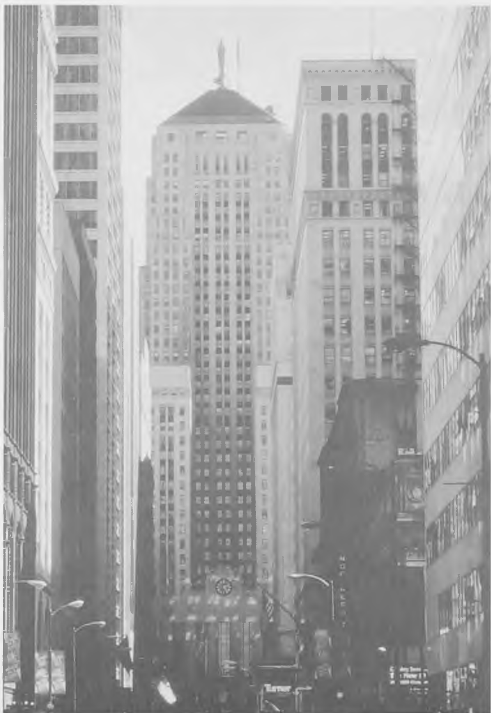
La Salle Street – Board of Trade Building
