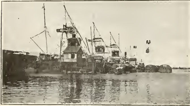
FLOATING DOCKS AND AERIAL CABLES.
