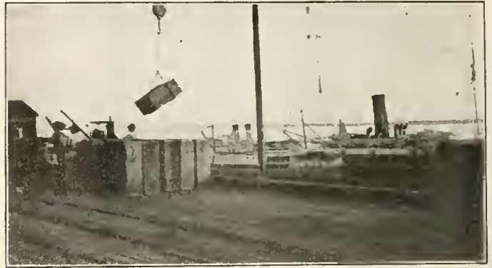
MOVING CASES OF RUBBER BY AERIAL CABLES.
