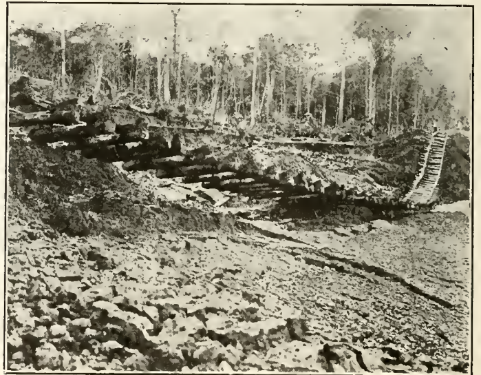
FILL AT STATION 54.
