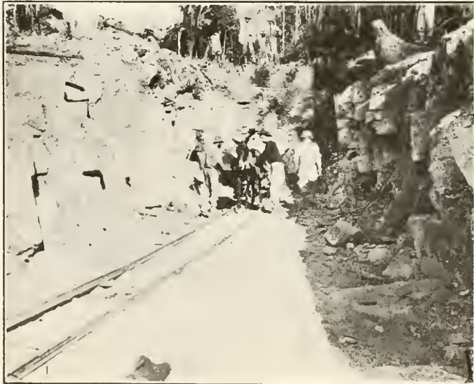
ROCK CUT ON RAILWAY LINE.
