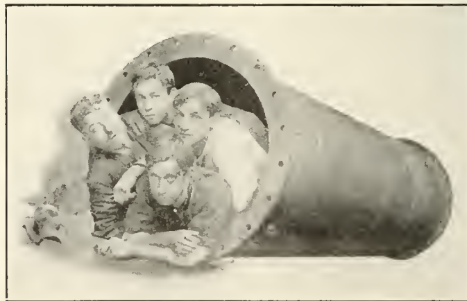
A LARGE SECTION OF DREDGING HOSE.
