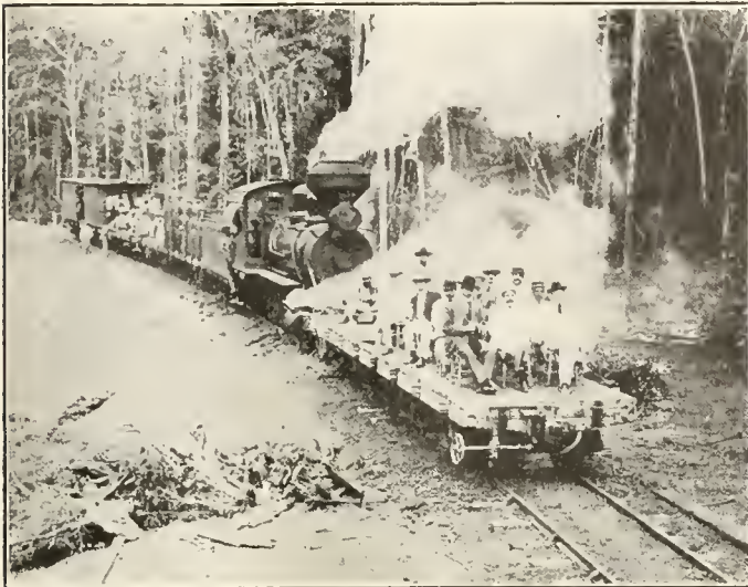
CONSTRUCTION TRAIN ON THE MADEIRA-MAMORE.
