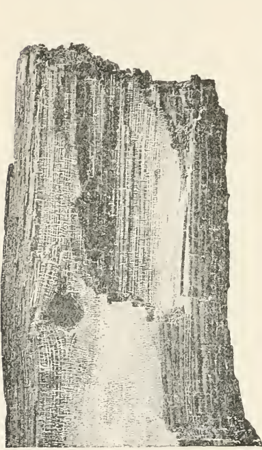
FIG. 270.— Polyporus borealis . Destruction of Spruce-wood. The white mycelium is present, dividing the decayed wood into cubical pieces. (v. Tubeuf phot.)
