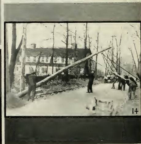
8. PULLING AERIAL CABLE WITH WINCH. 9. PULLING UNDERGROUND CABLE WITH WINCH. 10. SEALE AND WARRINGTON LAY WINCH ROPES. 11. TRACTOR CABLE PULLER. 12. CAR UNLOADER. 13. UNLOADING 5-TON REEL OF CABLE. 14. PIKING IN A POLE.
