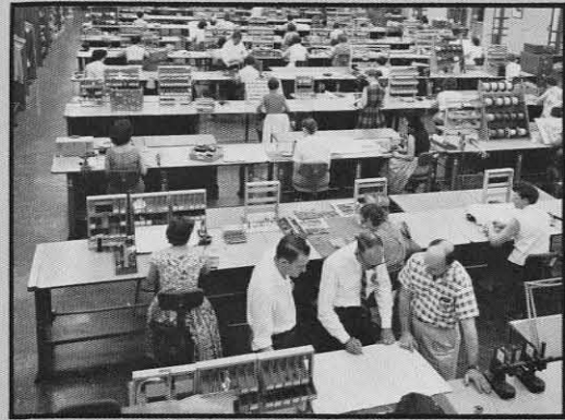
Production of communications equipment in new Los Angeles manufacturing plant
