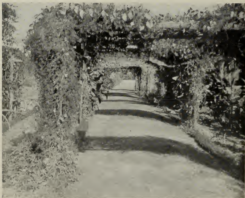
FIG. 195.—THE PERGOLA, LOOKING NORTH.
