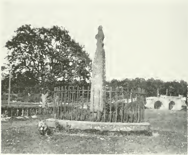
Boatford Cross and Nith Bridge
