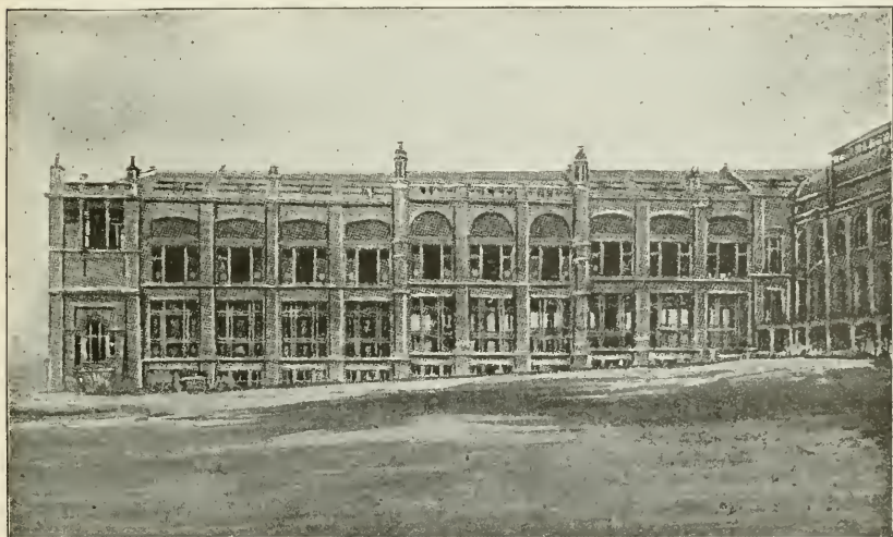
FIG. 115.—Royal Museum of Natural History, Brussels, Belgium. One of the long sides of the building.
