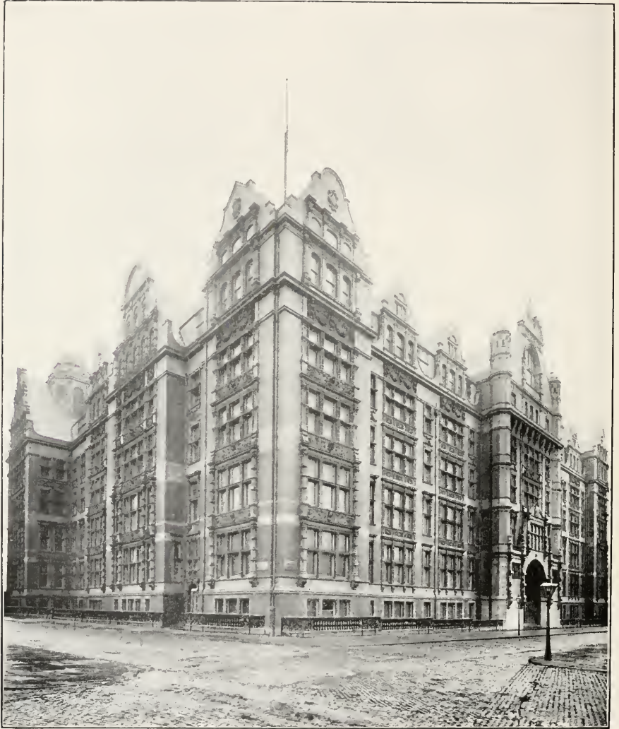
MUNICIPAL TECHNICAL SCHOOL. Manchester, England.
