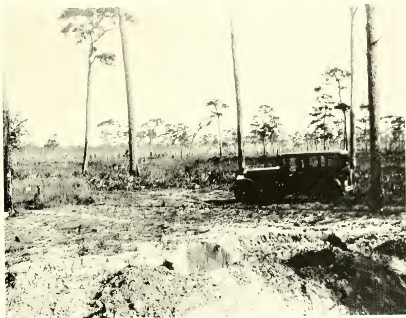
1. General view of the Seminole area with excavation in foreground. Photograph by W. W. Holmes.
