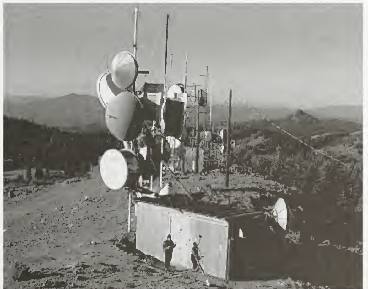
Fig. 2) View of communication facilities from Soda Mtn. Lookout. View is looking down main ridge (SW). Pilot Rock on right.
