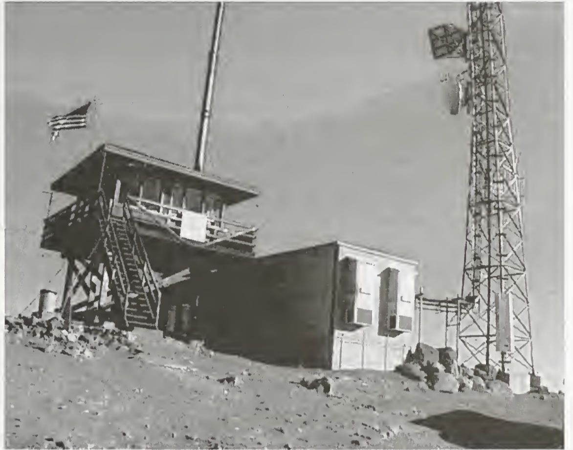
Fig. 1) View of Soda Mtn. Lookout owned by Oregon Dept. of Forestry. Communications building and tower owned by AT&T Wireless.
