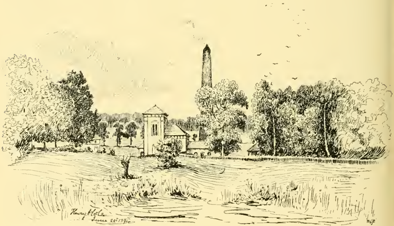
RYE COMMON PUMPING STATION, NEW RIVER COMPANY, ST. MARGARET'S, HERTS., SEEN FROM THE LEA.
